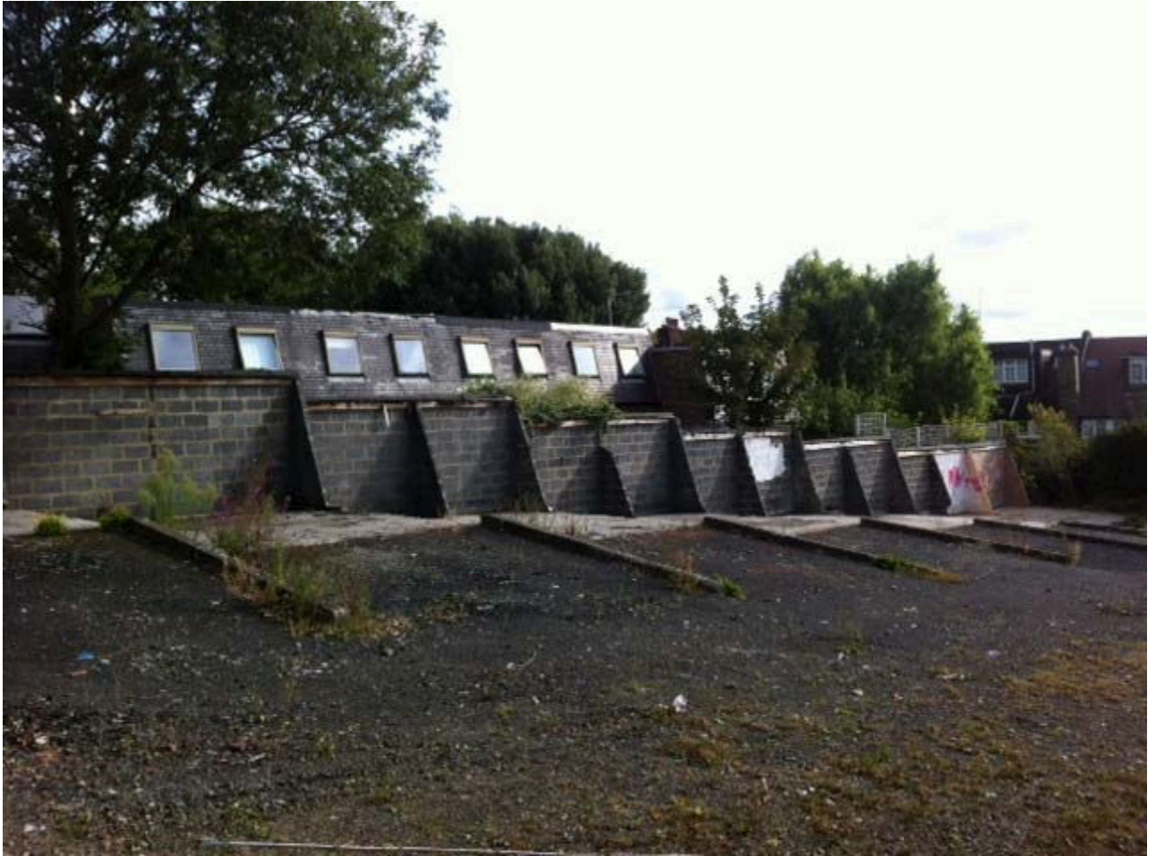
Northern Boundary Wall of Site
